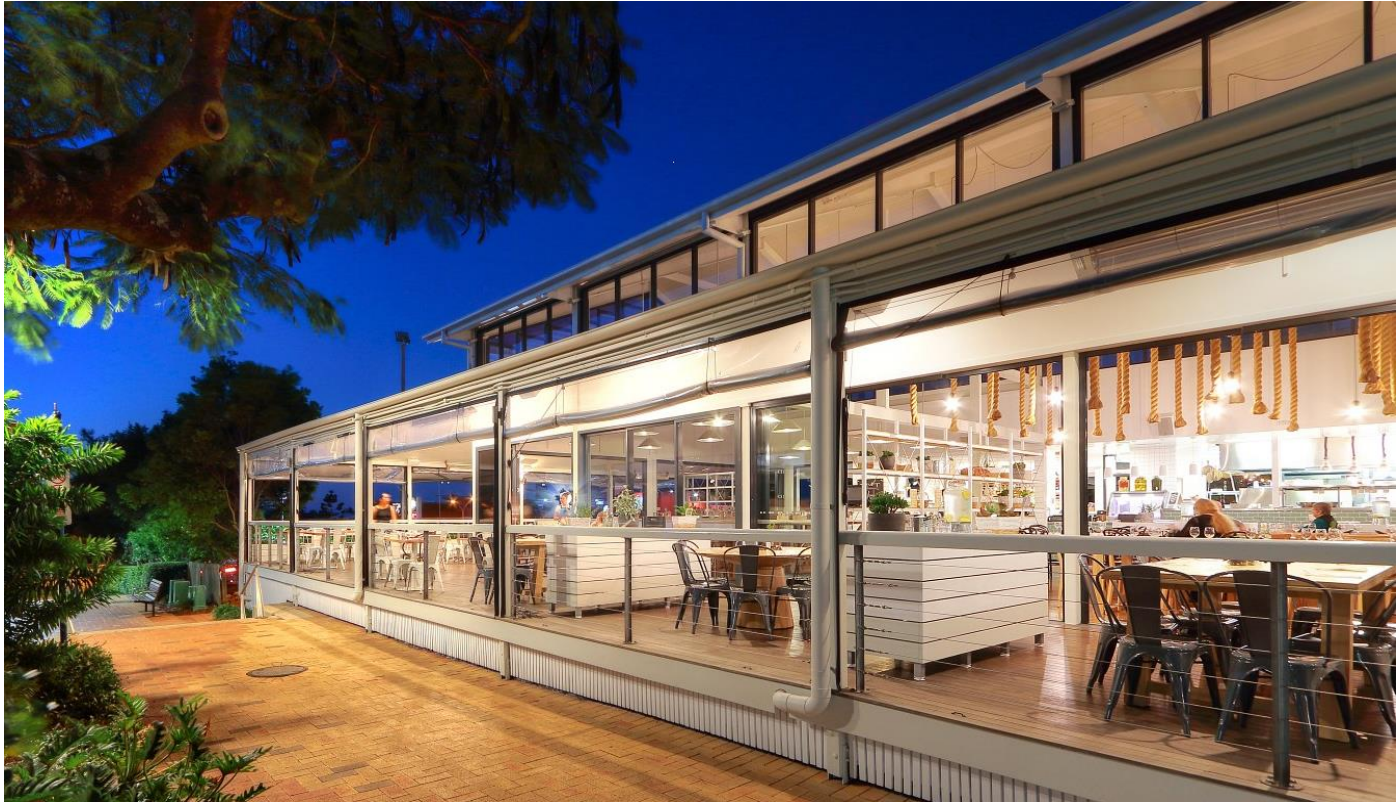
Al Fresco dining refurbishment, The Cleveland Sands Tavern, Cleveland, Brisbane
